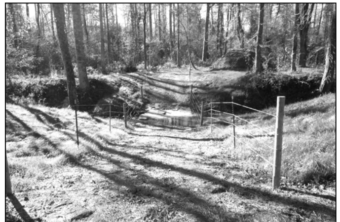
A stream crossing that limits access and protects the rest of the buffer.
